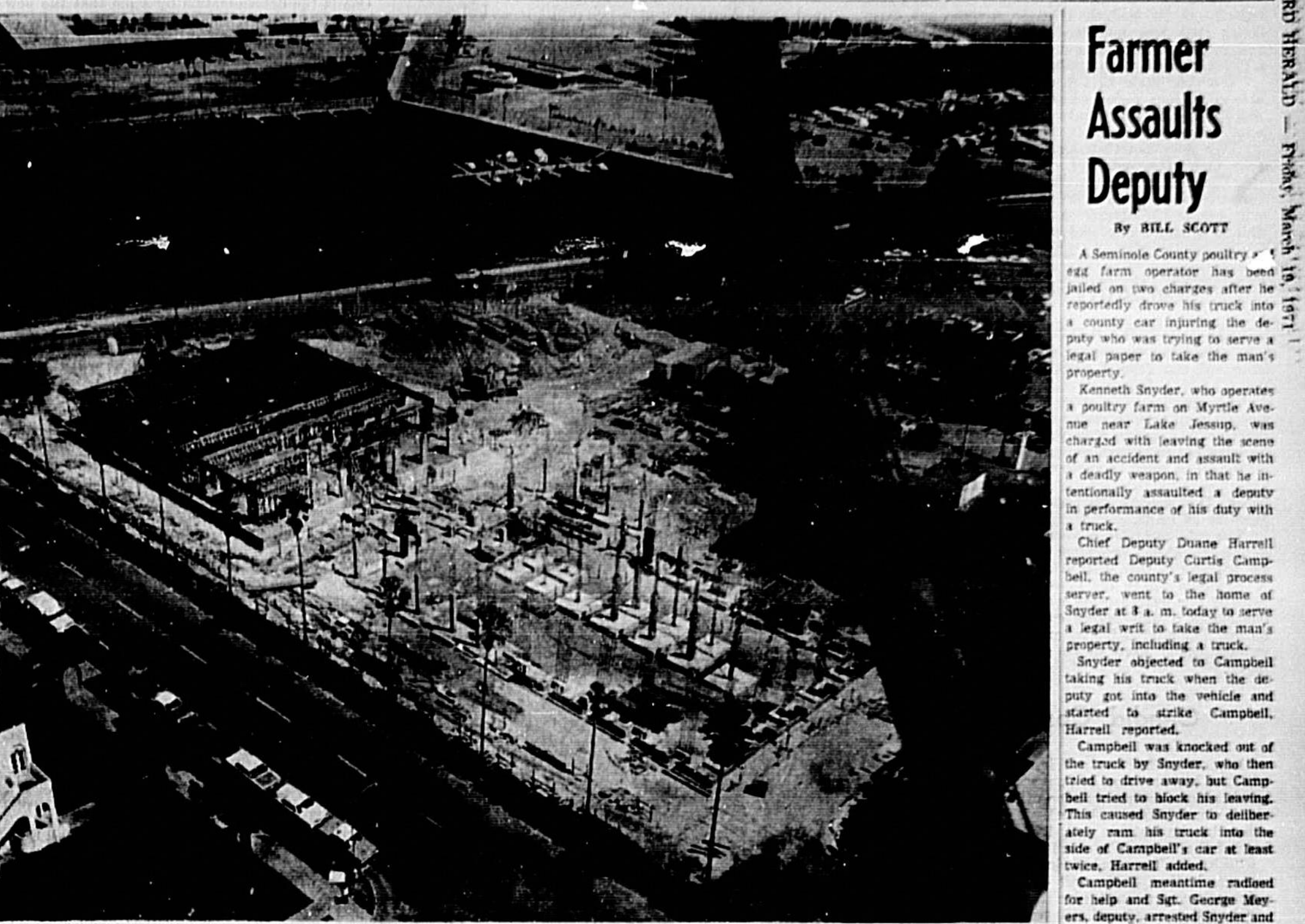
Progress photo of Seminole County's new $4.2 million court house, slated for occupancy in the Spring of 1972. West harbor of Holiday Isle marina at top; Sanford city hall at lower left, and county jail at right center. (Aerial Photo by Bill Vincent Jr.)
