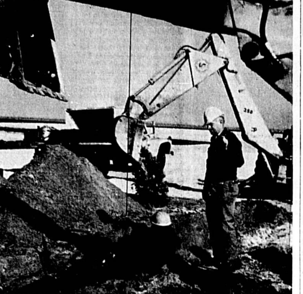
WORK ON LAYING water lines into the massive Marina complex got underway yesterday afternoon. Shown above is City Manager W. E. Knowles supervising the project. Knowles said this morning it would take close to a week for the lines to be tied in. (Herald Photo)
