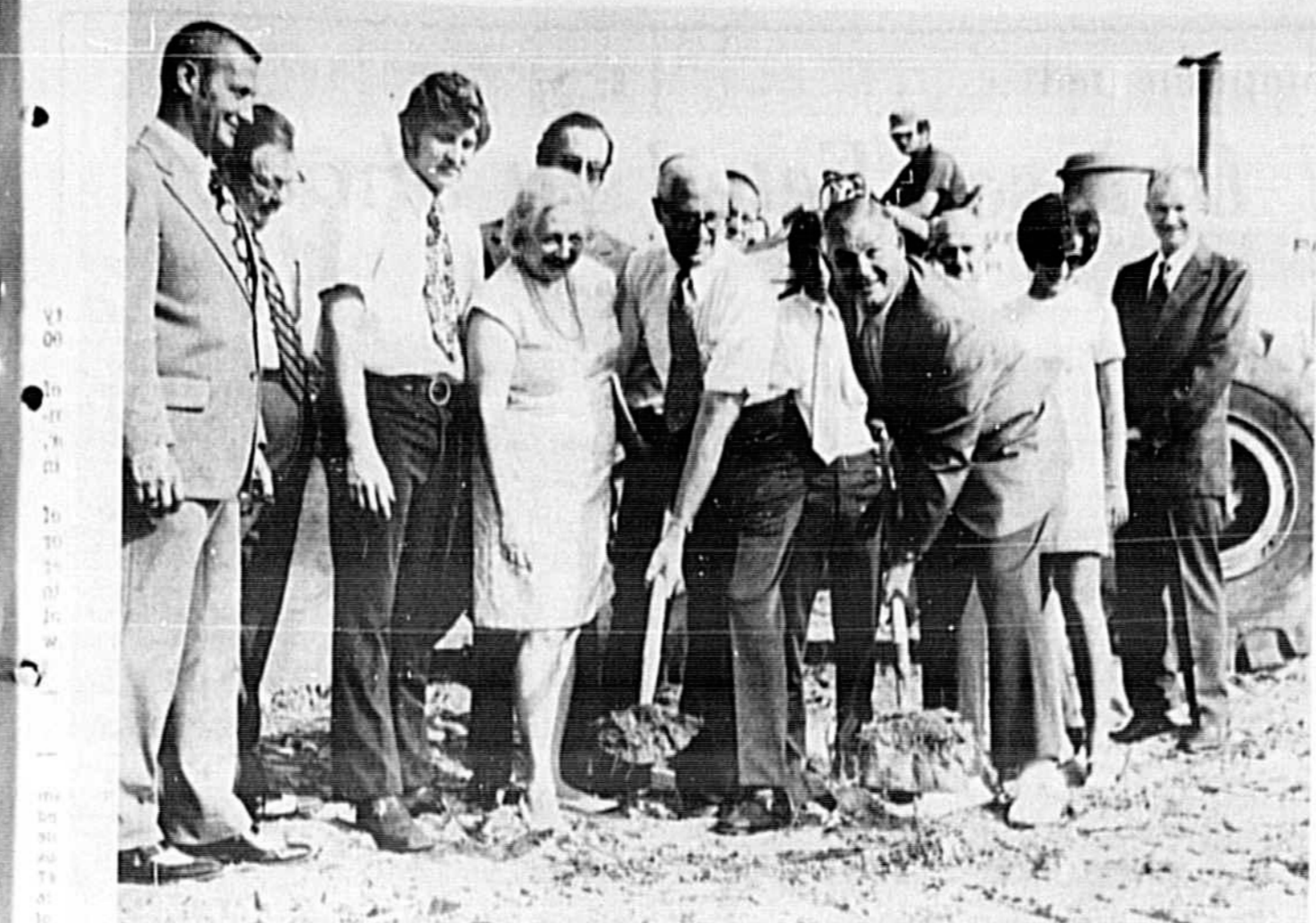
GROUND is broken for the new $100,000 steel facility to house Southern Shortenings on County Club Road. Breaking ground are Dr. and Mrs. George Jackson, owners of the company, assisted by Mayor Lee P. Moore. The
