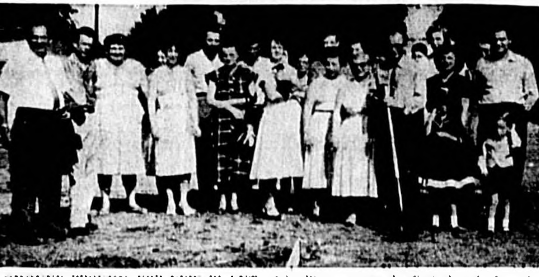
GROUND BROKEN FOR NEW PLANT—John Pietro turns the first shovel of earth at the site where the new Pietro Manufacturing Co. plant will be erected. At extreme left is John Kridler, manager of the Seminole Chamber of Commerce. Mrs. Pietro is immediately to the left of her husband. Watching the Saturday ceremony were employees and others who attended. (Photo by Bergstrom)
