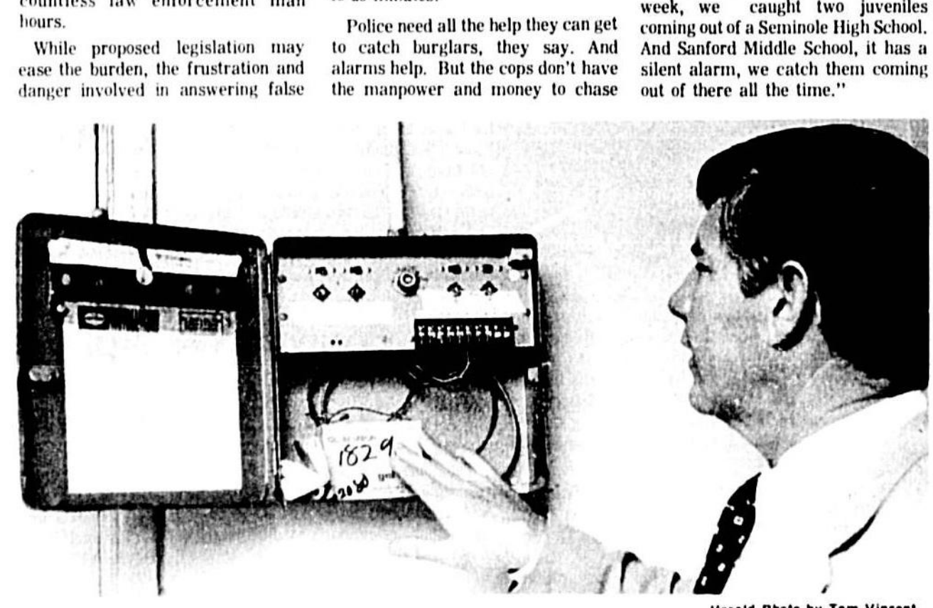
Sanford Middle School Principal Dan Pelham shows the school's burglar alarm panel which has been credited in the apprehension of many school burglars.
