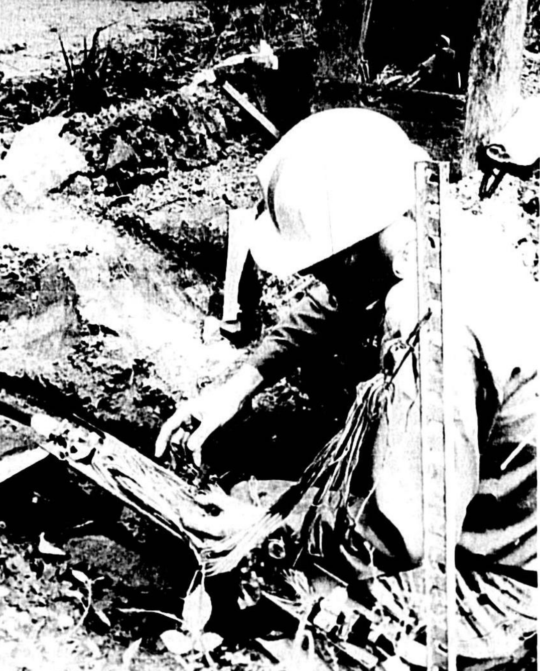
Don Oliver installs new cables near Oviedo
