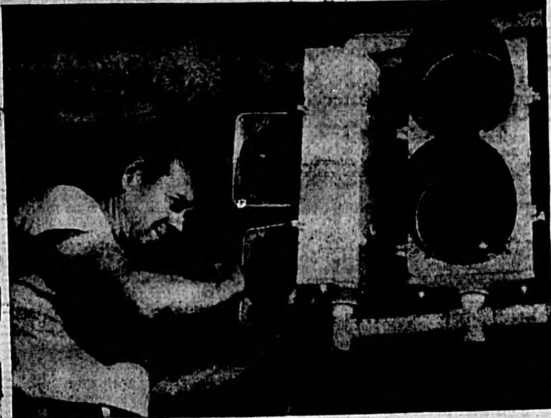
WAIT AND WALK LIGHTS are now in operation at First St. and Park Ave. Don Young of Sanford Electric Co. puts finishing touches on the synchronized system yesterday. Pedestrians can walk four ways with safety. Now that the new lights are operating. (Photo by Bergstrom)
