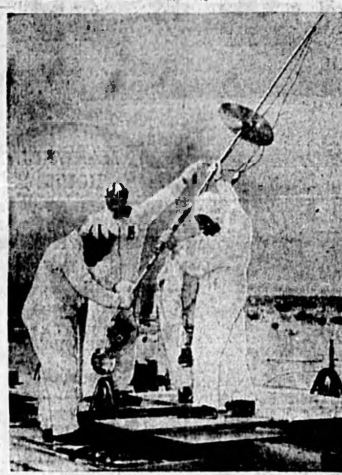
THEIR POSE MAY RECALL the historic two Jima flag-raising incident, but the scene is the Sanford atomic plant at Richland, Wash., and the men are General Electric Company technicians who created their odd-looking equipment for taking pictures inside underground storage tanks for radioactive waste. The device they are raising is a steel "fish pole" on which is mounted a camera that can get photos in a tank that has only a nine-inch entrance. The disc serves to block escape of radiation while pictures are being made. (International)
