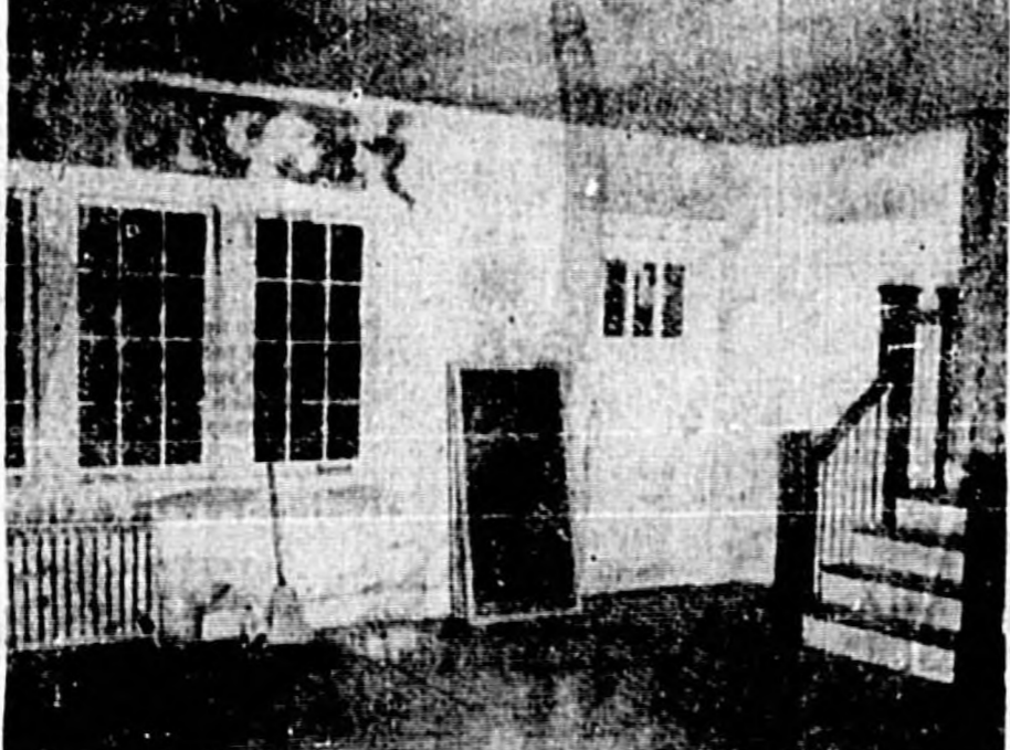
BEFORE "Do-It-Yourself!" Carlton tackled his project, the living room looked like this. He had to sweep up fallen plaster from the floor. But he knew he had sound construction—an oak floor here.
