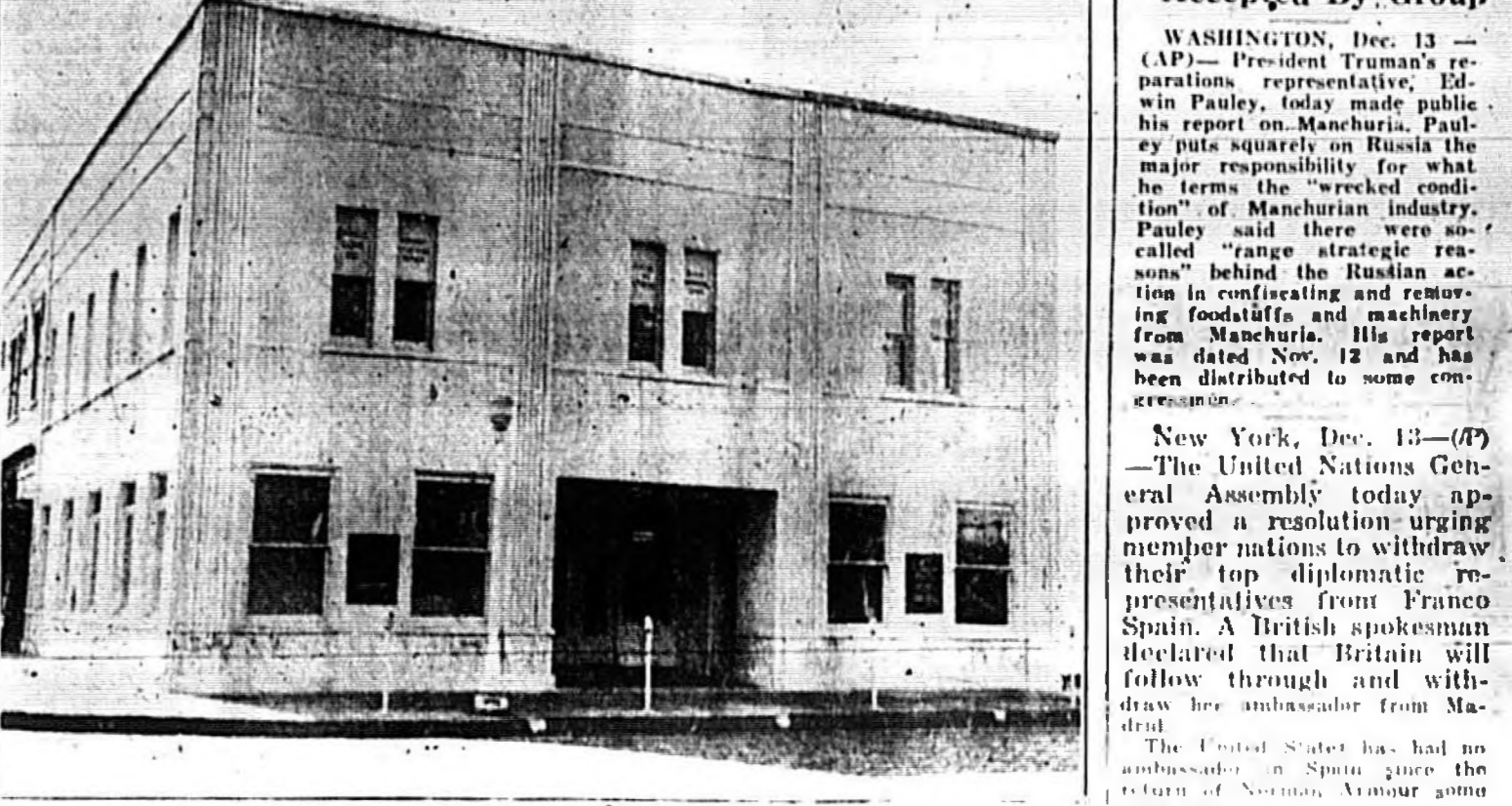
The Florida State Bank building at Park Avenue and First Street is shown as it now appears after it was renovated with a new bank entrance placed with office space on either side, and the old marble exterior replaced by white stucco. The new sign for the front of the bank has not yet been completed.
