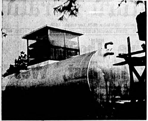
**CASSELBERRY UTILITIES** has completed improvements at the South Pump, pictured, including new aeration tanks, aerator, chlorinator and pump and construction has received certification from the engineer. Water analysis have been approved by the State Board of Health and the town is now being supplied from this pump while the 100,000 gallon storage tank at the main pump is being completed. (Herald Photo)
