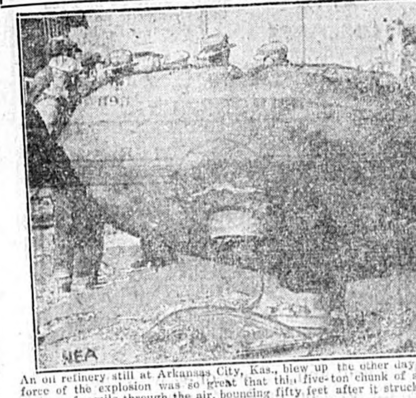
An oil refinery still at Arkansas City, Kas., blew up the other day and burned three men to death. The force of the explosion was so great that this five-ton chunk of steel on top of the still was thrown a quarter of a mile through the air, bouncing fifty feet after it struck the ground.
