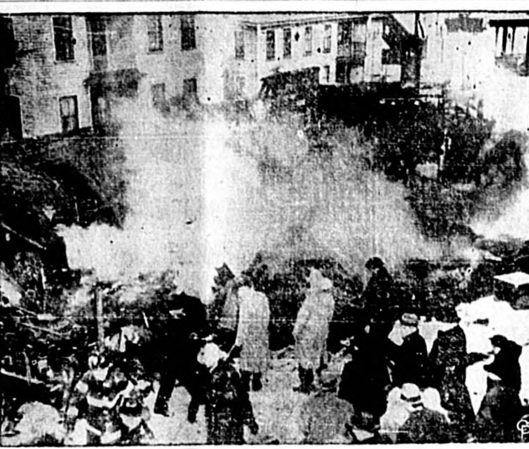
ELEVEN members of one family perished in a flash fire that swept a two-story frame home (above) in Utica, New York. Firemen and rescue workers are shown around the collapsed building. Ten bodies were recovered by firemen from the smoldering ruins. Eight were those of children. One was that of a woman, clapping an infant. Fourteen severely ill persons fled from the building. Those persons were hospitalized with burns after jumping from a second-floor window. (International photograph)
