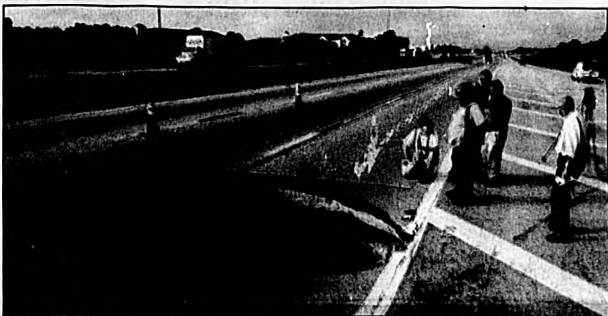
Department of Transportation employees inspect a sinkhole on Interstate-4. The geological phenomenon emerged Wednesday morning and was first reported by a passing motorist. Pictured at top, traffic was backed up for 8 miles after all but one of the westbound lanes near the Lake Mary exit were shut down following the first reports of the sinkhole.
