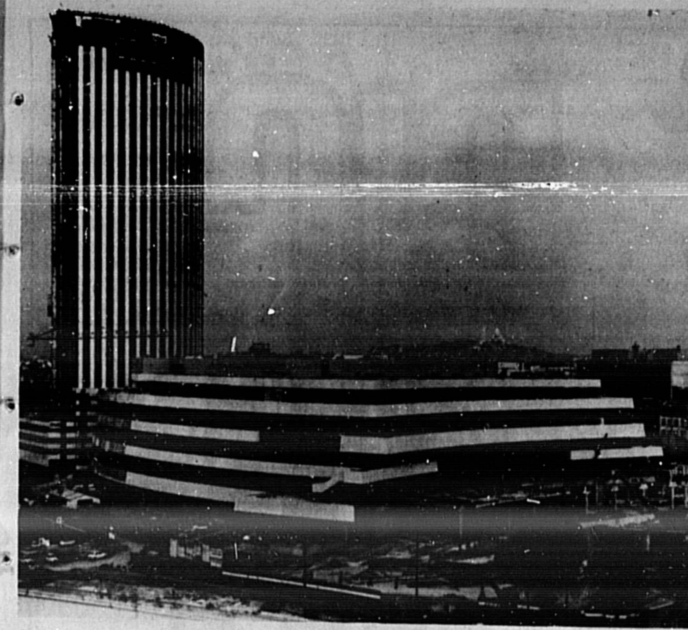
HIGH-RISE IN PARIS ...Cost $100 million
