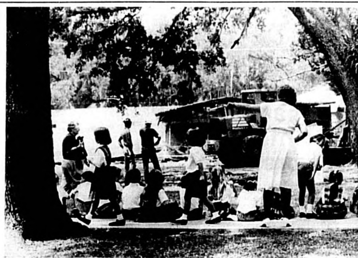
Playtime for children at All Souls Catholic School this week included watching workers demolish an old classroom. The building, built in 1954, is being replaced by a new facility on the school grounds near 9th Street and Oak Avenue.
