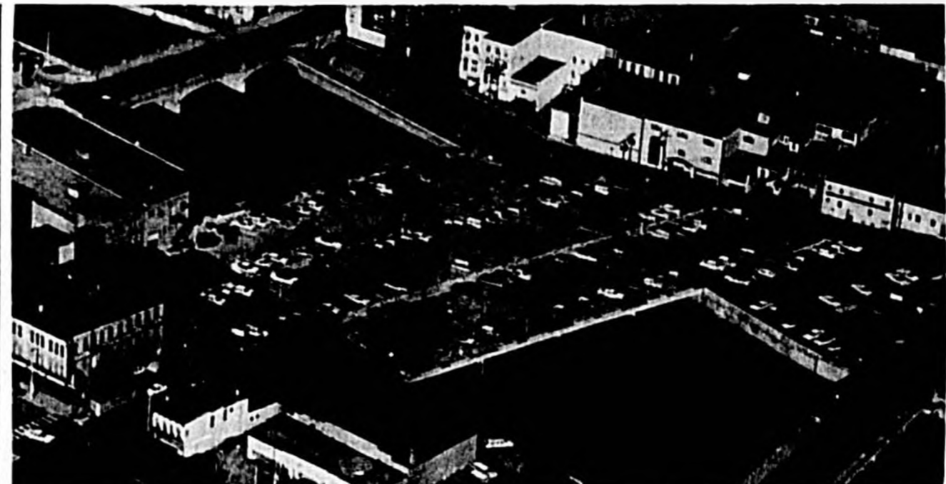
SANFORD CITY officials could take a hint from Janesville (Wis.) in finding space for municipal parking lots. For decades Rock River had split Janesville. Today the river no longer divides the city. A parking plaza sits astride the river (pictured above) and has revitalized the downtown area. Sanford officials could well build
