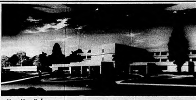
Construction is moving forward at a good clip on the $30 million South Seminole Medical Complex on a 26-acre tract north of State Road 424 and west of County Road 427 in Longwood.
