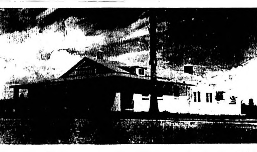
The above photograph of the new Recreation Building for citizens, now which will be dedicated Wednesday at 2:30 P.M. and turned over to the National Catholic Community Service, was taken by an official photographer of the Sanford Naval Air Station. M. W. Langer, P.M.
