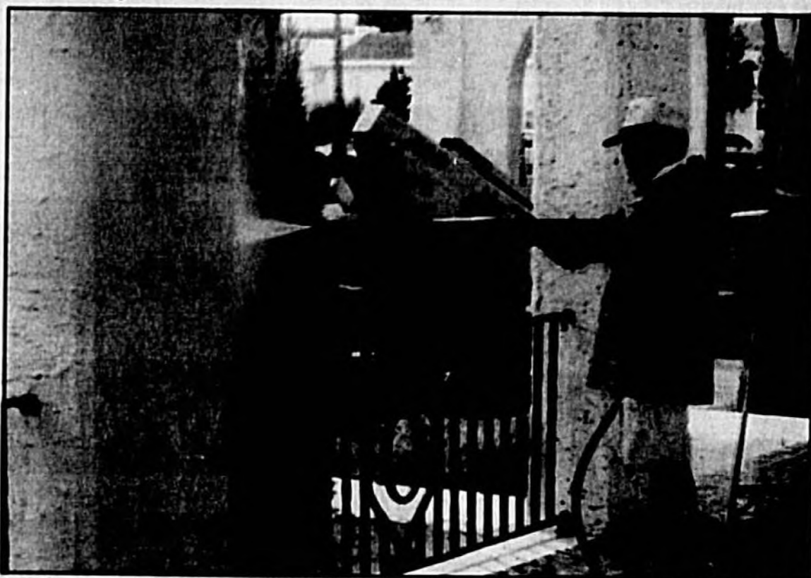
Tony Rico of Cine's Painting in Sanford pressure cleans old paint off the New Tribes Mission Headquarters Building on East First Street in Sanford. The building is in the process of receiving a new coat of paint. The outside color will change from white to a light tan. Herald photo by Art Simmons
