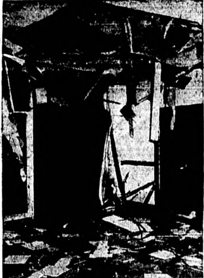
BLAST WRECKS NASHVILLE JEWISH CENTER—The lobby of the Nashville, Tenn., Jewish Community Center hangs in shreds after a dynamite blast rocked the building. A similar blast a few hours earlier had heavily damaged a Jewish center in Miami, Fla., but it was not known if the two incidents were connected. (UP Telephone)
