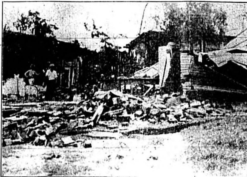
Four persons were killed, thirty or more were injured and heavy damage was done to property when the second hurricane of the season tore through sections of Cuba. This picture shows the splintered ruins of buildings in the Santiago region. (Associated Press Photo)
