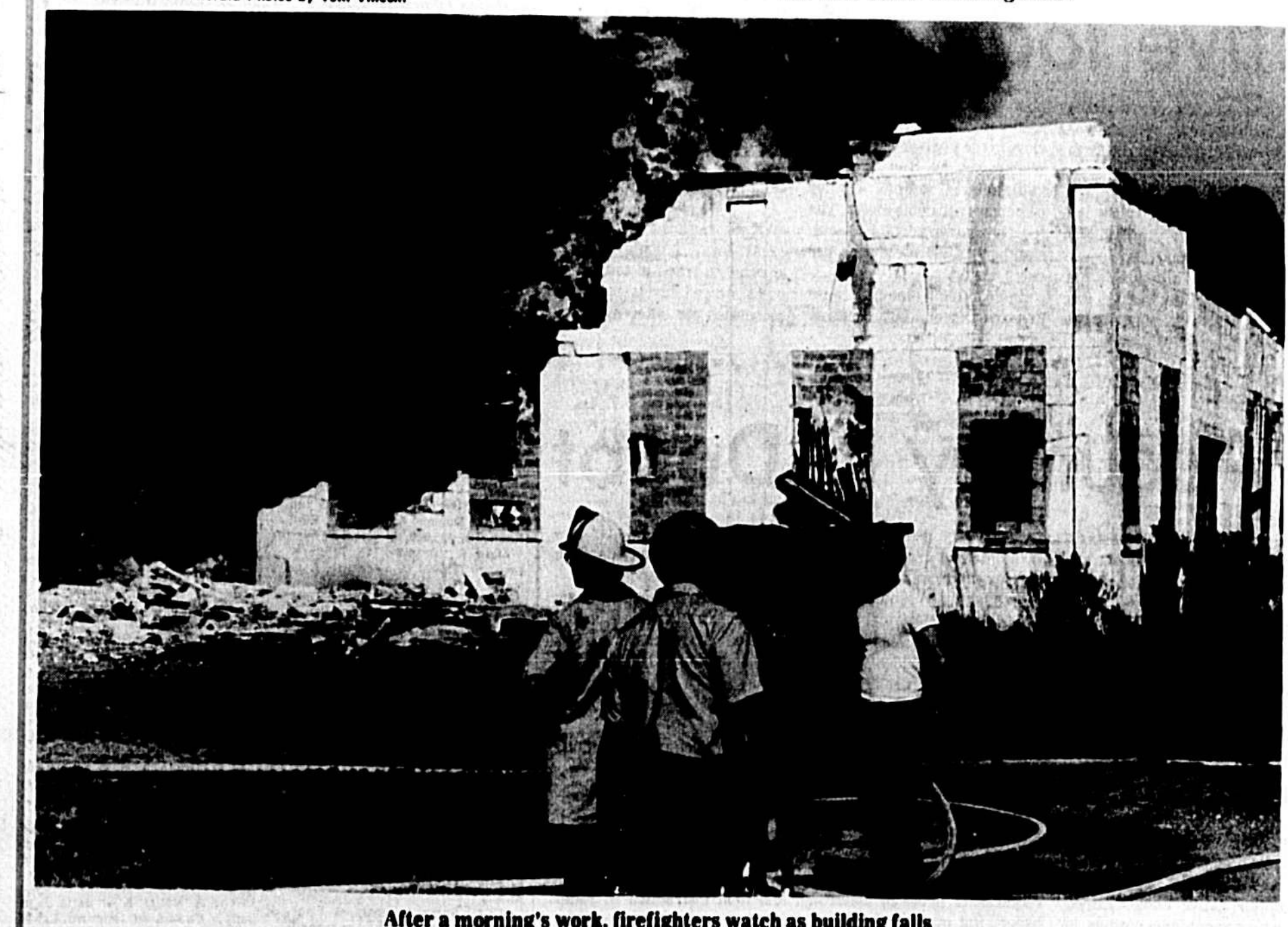
After a morning's work, firefighters watch as building falls
