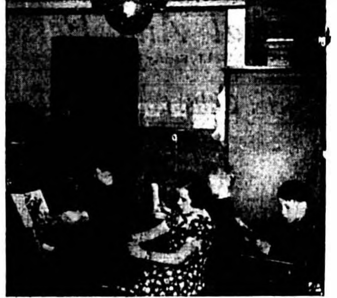
GERM-FREE AIR for school pupils is goal of University of Pennsylvania scientists directing installation of a new lamp in this junior grade room at Germantown Friends school. From the lamp, invisible ultra-violet light radiates, cleansing the atmosphere—it is believed—of harmful bacteria.
