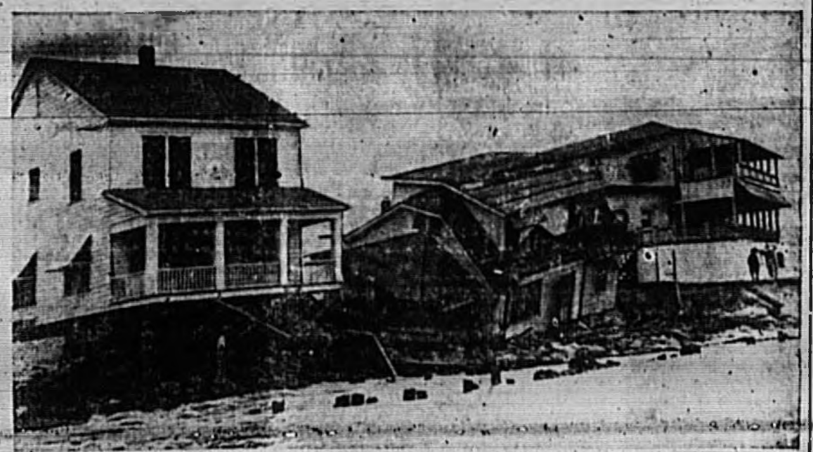
THESE TWO HOUSES WERE WRECKED at Smyrna Beach, Fla., after a flash storm at sea off the northeastern coast of Florida caused excessive high tides. Numerous homes and buildings along the State's beach-fronts were damaged. In the area near Jacksonville damage was estimated at about $300,000. (International)
