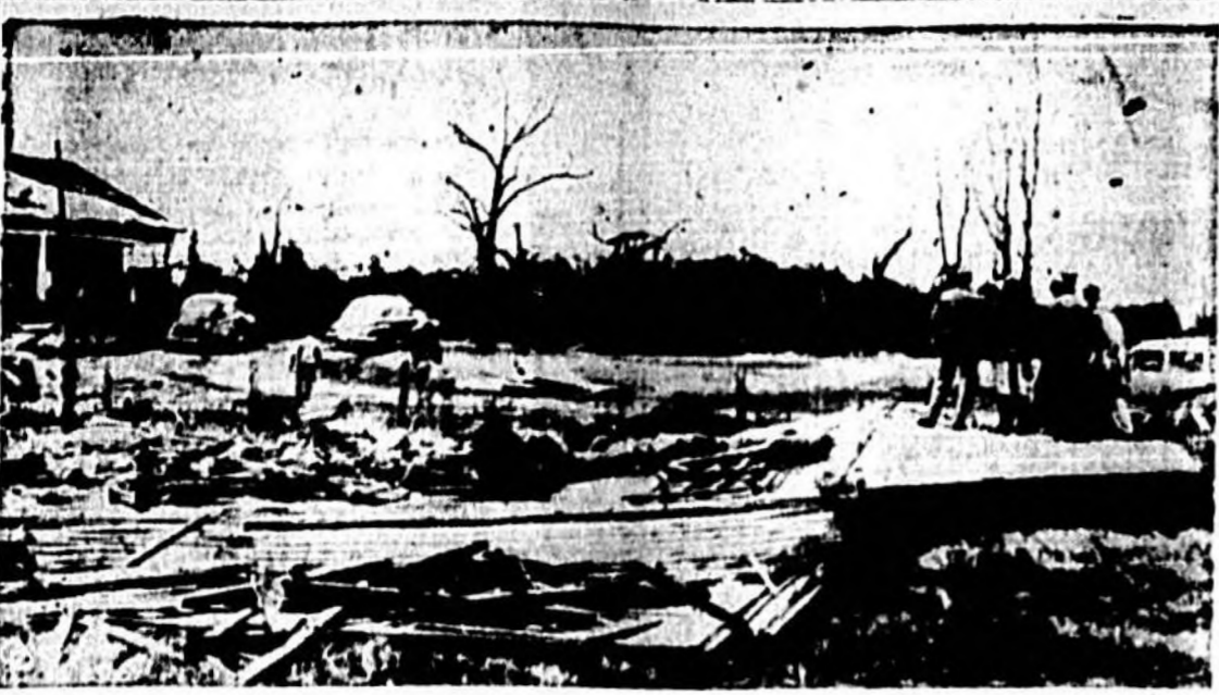
THIS WRECKED PLANTATION NEAR YAZOO CITY, MISS., was in the path of "snork" hard-hitting tornadoes that cut a crazy-quilt pattern across Georgia, Mississippi, Kentucky and Louisiana. Seven persons were killed and 21 others were injured in the Yazoo County area. Heavy rains accompanied the twisters and Red Cross crews were struggling through mud to perform rescue and rehabilitation work. (International Soundphoto)
