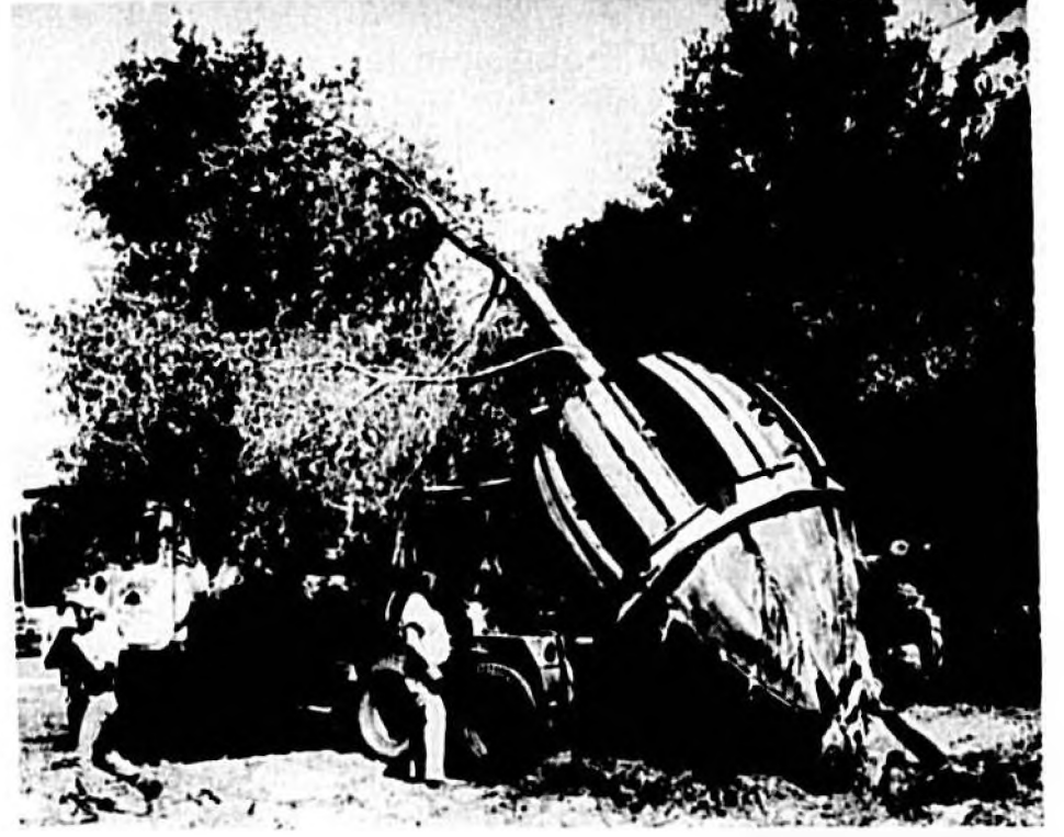
Daniel Wester (left) and Don McLaren hoisting trees saved from Lake Mary Boulevard widening project.
