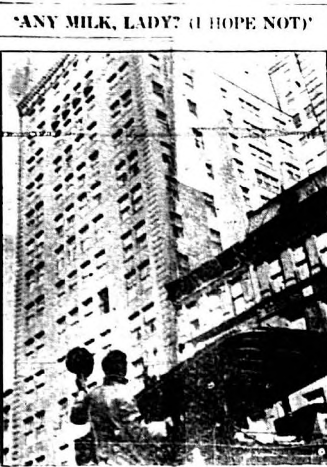
The life of the building who has been completed, very early in the New York work on the top of the building. It is now being built as though it were a skyscraper.
