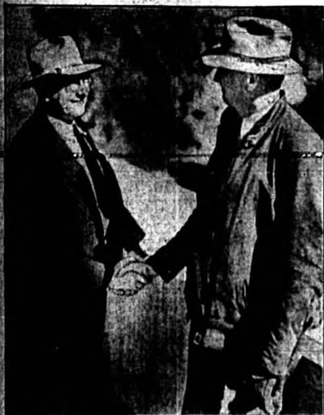
"Hard rock" engineers don't go in very much for formality—and so the great Boulder Dam on the Colorado river was delivered to the United States government by the contractors with no more ceremony than a handshake. "It's yours," simply exclaimed Frank Crowe (right), superintendent for the builders, as he greeted Ralph Lawry (left), engineer representing the federal reclamation service, upon completion of the gigantic project. (Associated Press Photo)
