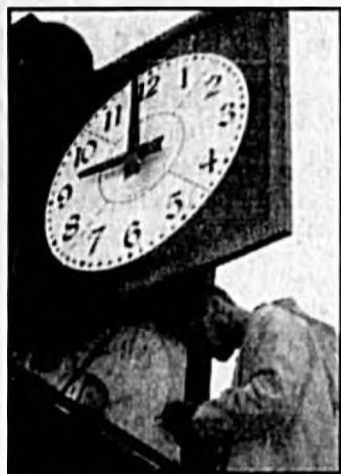
Shawn Wood of Palmer Electric installs new works in the clock.
