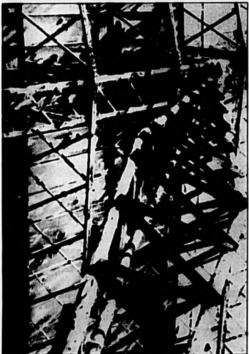
The intricate skeleton behind the Movieland Drive-in screen.
