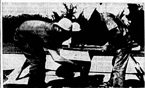
CITY CREWS installed base standards Wednesday for poles which will hold new traffic signal light at the corner of Oak Ave, and First St. Traffic signals are expected to relieve congested area on this corner.
