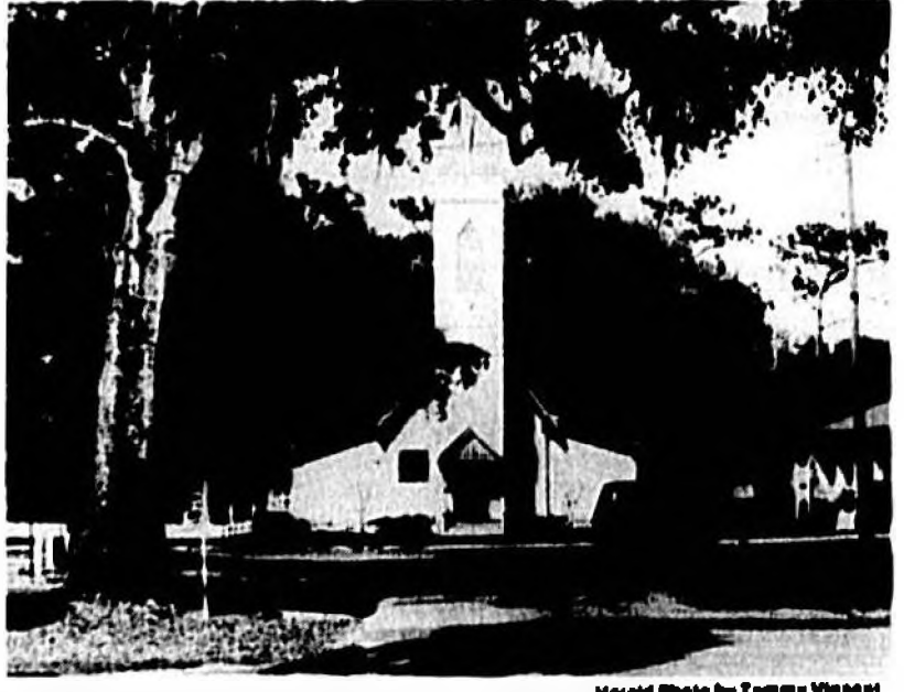
A historic Episcopal church in Longwood. Photo by Tommy Vincent
