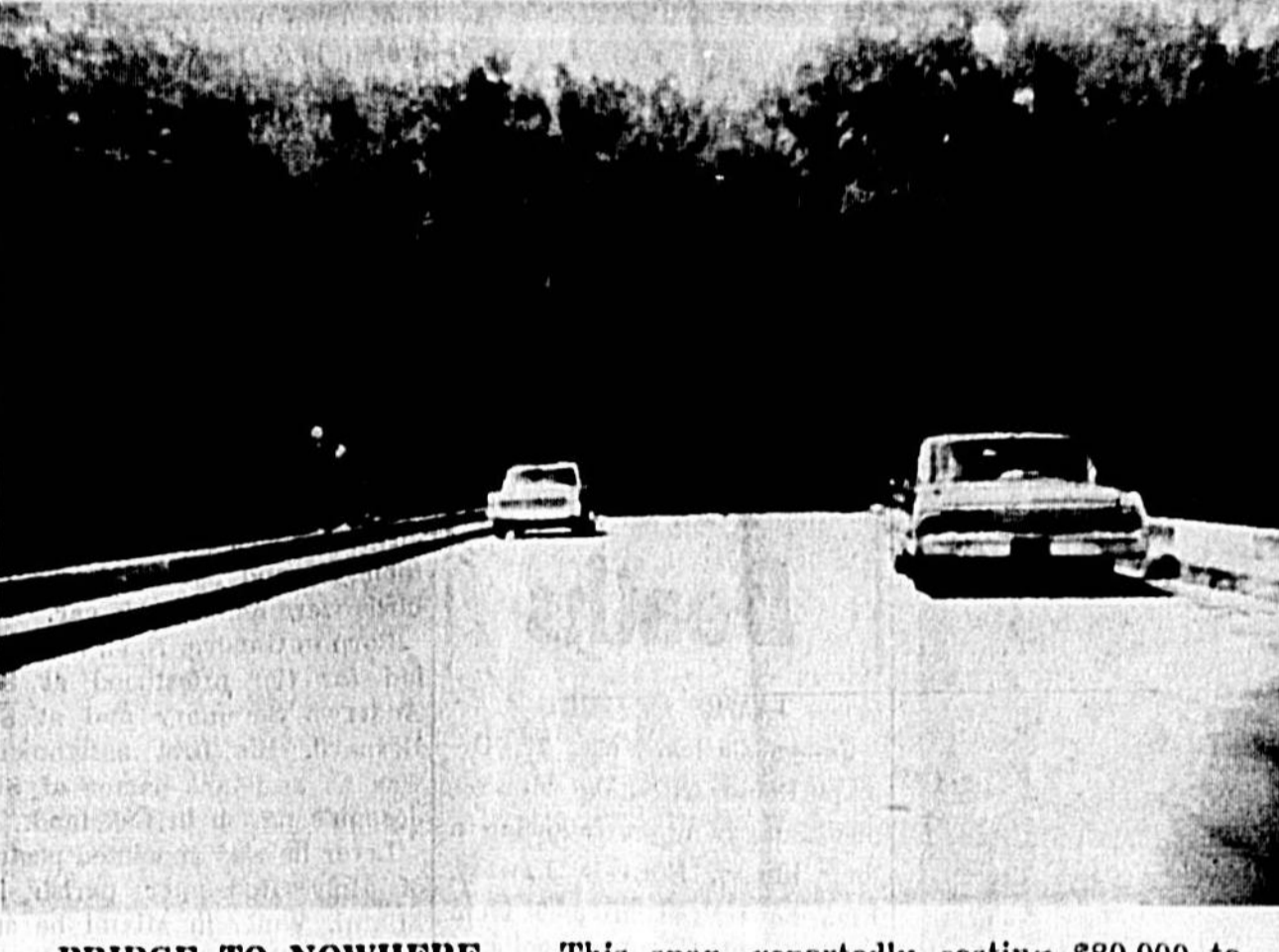
BRIDGE TO NOWHERE — This span, reportedly costing $80,000 to build 8-10 years ago, connects Seminole and Orange Counties, across the Wekiwa River. . . only motorists hit a wall of trees and weeds at the Orange end of the bridge. Road across the bridge, so 'tis said, was to connect with a new dead-end highway running south from SH 46 in Lake County. Span was built with private capital. State study of a recreation park in the area has revived the thought of completing the road to connect Lake, Orange and Seminole Counties across the Wekiwa River. (Herald Photo)
