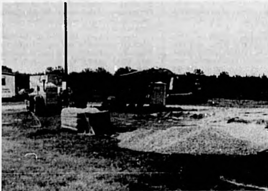
Town Centre Apartments is being built on West First Street, Sanford.
