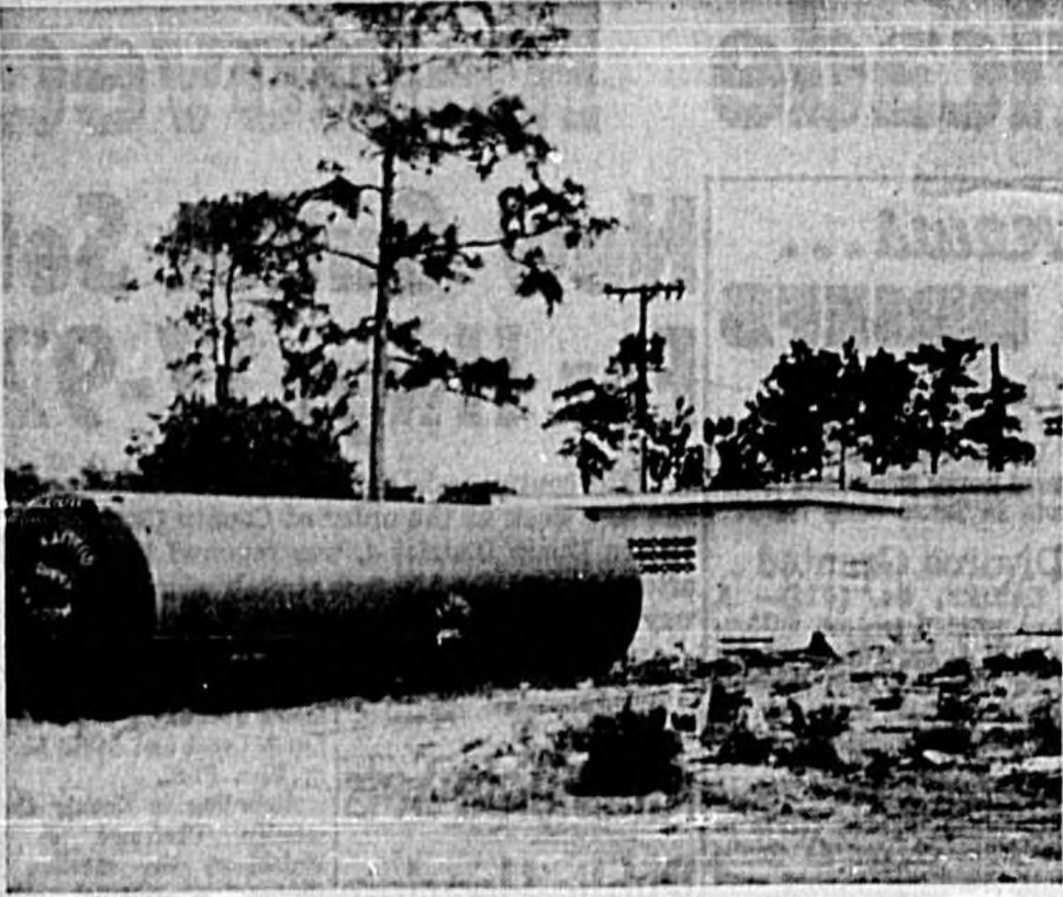
A NEW MODERN WATER PLANT is nearing completion in Chuluota with the water tank and piping expected to be ready for use within the next 30 days. Central Florida Utility Co., which is building the plant, will house an aerator system in the large building at the right. (Jones Photo)
