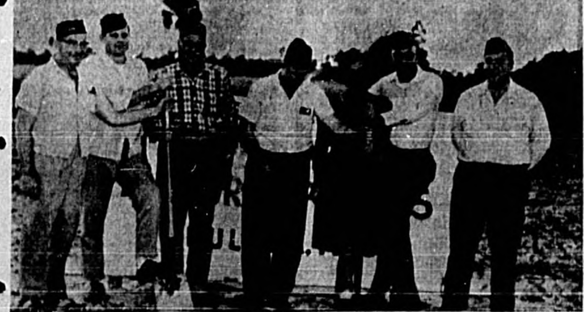
AMERICAN LEGION POST 225 of Chuluota broke ground for its future home in ceremonies last Saturday on the building site at the intersection of Christmas Rd. and Chuluota Rd. Taking part in the activities was Mrs. Edna Jacobs who donated the property to the Post which is named in memory of her husband. Others in the picture are, from left, Vincent Chambers, N. E. Runyon, Herbert Boswell, Wendell Jepson, Commander Ray Pentz and Ralph Warden. (Jones Photo)
