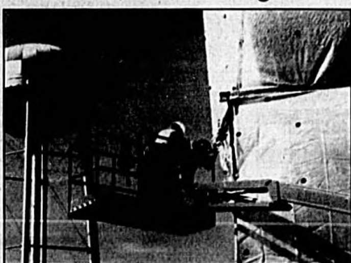
Employees with Goldman Painting and Sandblasting tape plastic sheeting around the Historic Sanford Memorial Stadium before beginning refurbishing. Herald photo by Tommy Vincent
