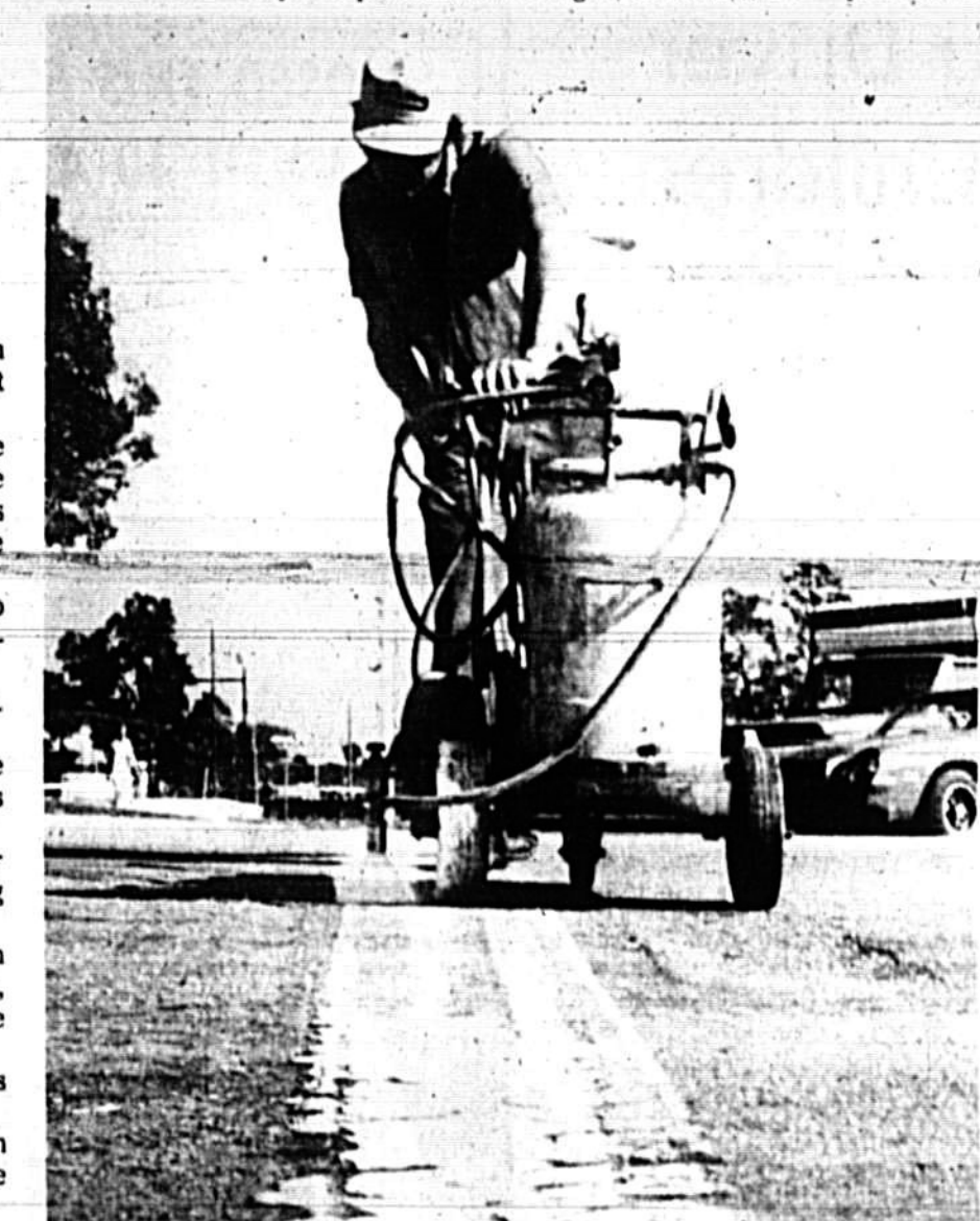
THE TRAFFIC STOPS HERE Sanford employee Glen Saunders spent Wednesday rewriting some old lines about the city. Sanford street department workers are repainting crosswalks and stop lines throughout the downtown area, including this crosswalk in front of the library. Sanford Photo by Tom Vincent
