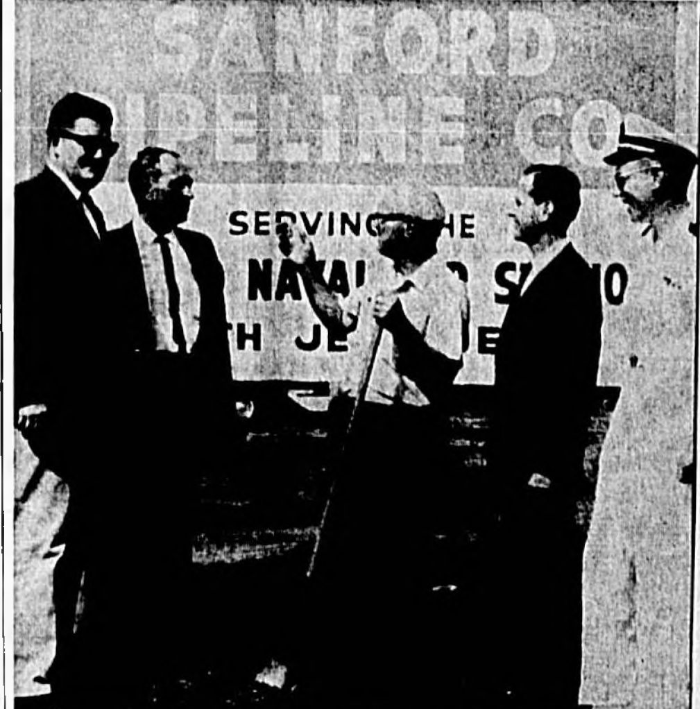
GROUND-BREAKING EXERCISES were held Wednesday afternoon for the new pumping station and storage tanks of the Sanford Pipeline Company at the lakefront adjacent to French Avenue. Plans are for the pipeline to be in operation within 90 days pumping Jet fuel from barges to the Naval Air Station. Pictured, from left: Mayor Tom McDonald, John Krider, Chamber of Commerce manager; Norris Plunk, pipeline superintendent; Gerald Rauch, president of Standard Southern Corporation, Houston, Texas, parent firm of the Sanford Pipeline Company, and Lt. Frank Wolfe, NAS assistant supply officer. (Herald Photo)
