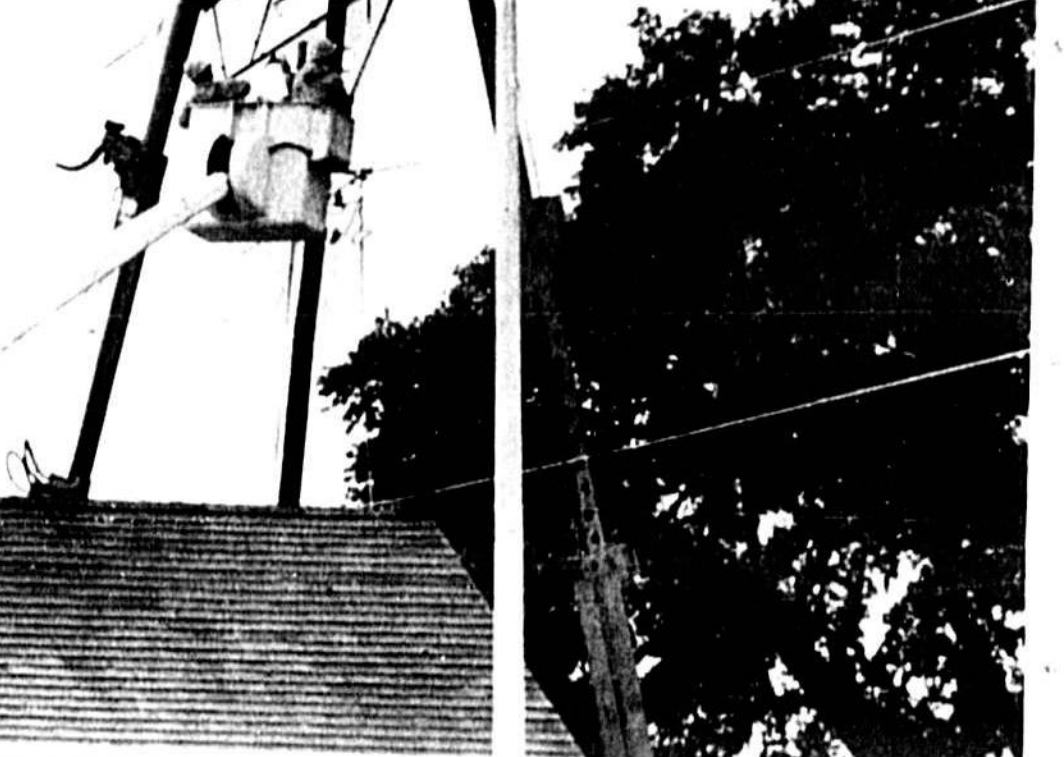
Florida Power & Light Company crewmen repair power lines at First Street and French Avenue in Sanford after violent thunderstorm struck area Friday afternoon, causing power outages.
