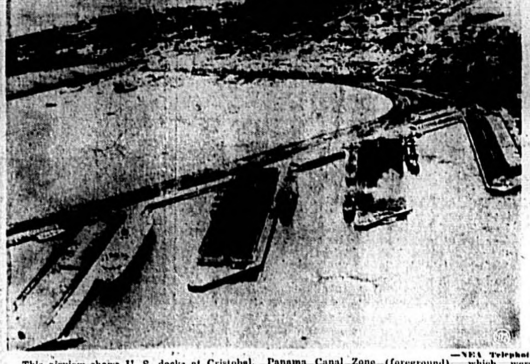
This airview shows U. S. docks at Cristobal, Panama Canal Zone (foreground), which were endangered by the fire that swept through Colon, making thousands homeless.
