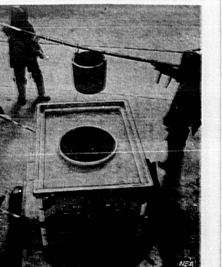
Armed-armed policemen in Pittsburgh, Pa., place suspected "bombs" in a fiberglass-reinforced container (left) and carry it to special stand-off trailer (right) where it will rest inside, larger, stiller one. Two-ounce bomb transporter, designed by JPG Industries, has convex bottom to direct force of blast upward.
