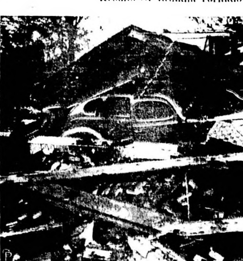
A GARAGE WAS NO PROTECTION for the family as a three-toned tornado smashed through Terre Haute, Ind. The walls were blown in and the ceiling collapsed on the table as the wind tore across the town. Forty-five persons were killed and 100 were injured in the town ripped from the Midwest states. (International)
