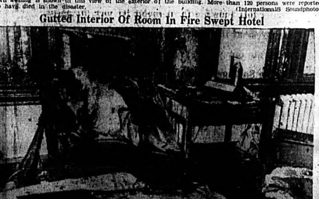
GUTTED INTERIOR OF ROOM IN FIRE SWEEP HOTEL
