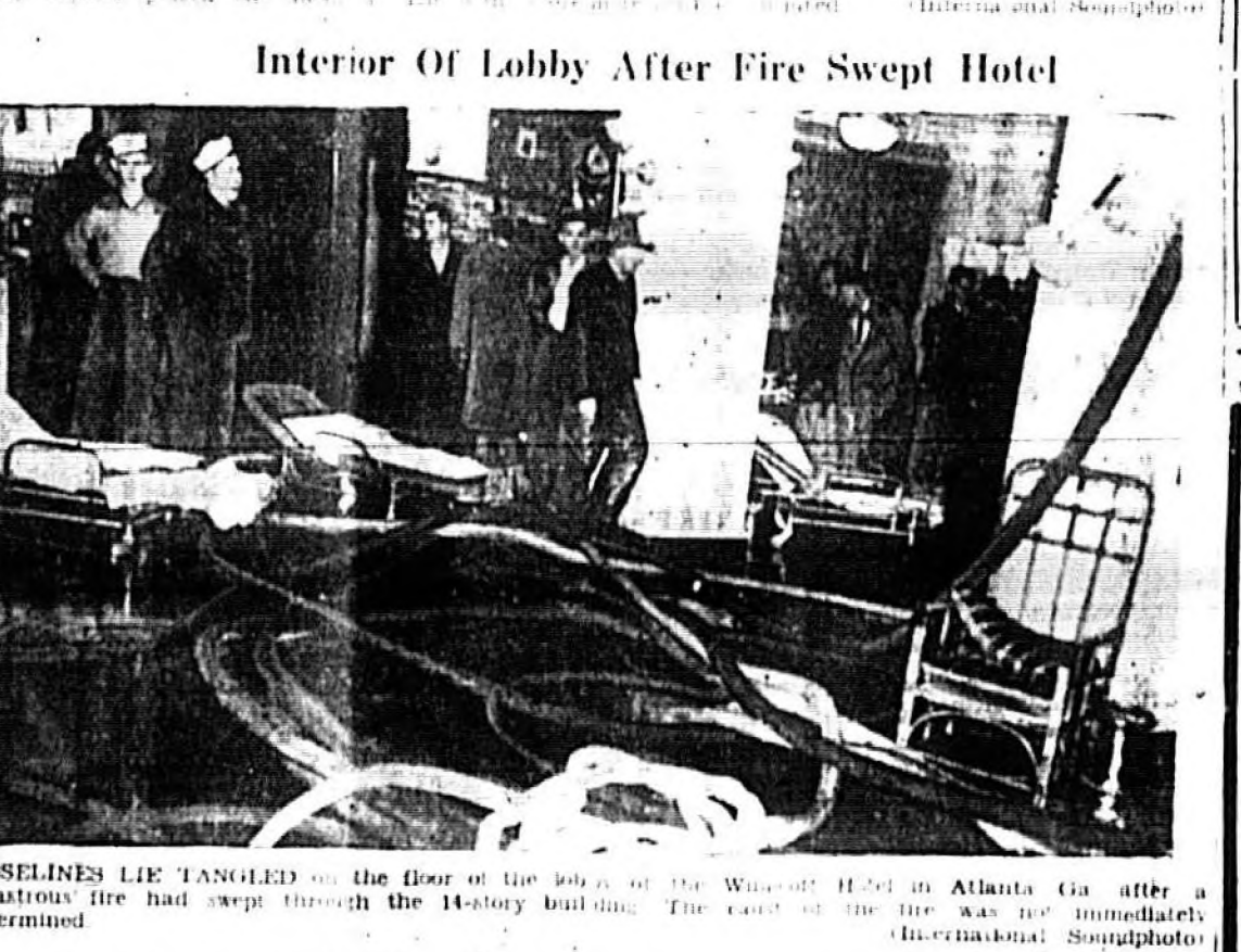
INTERIOR OF LOBBY AFTER FIRE SWEEP HOTEL
