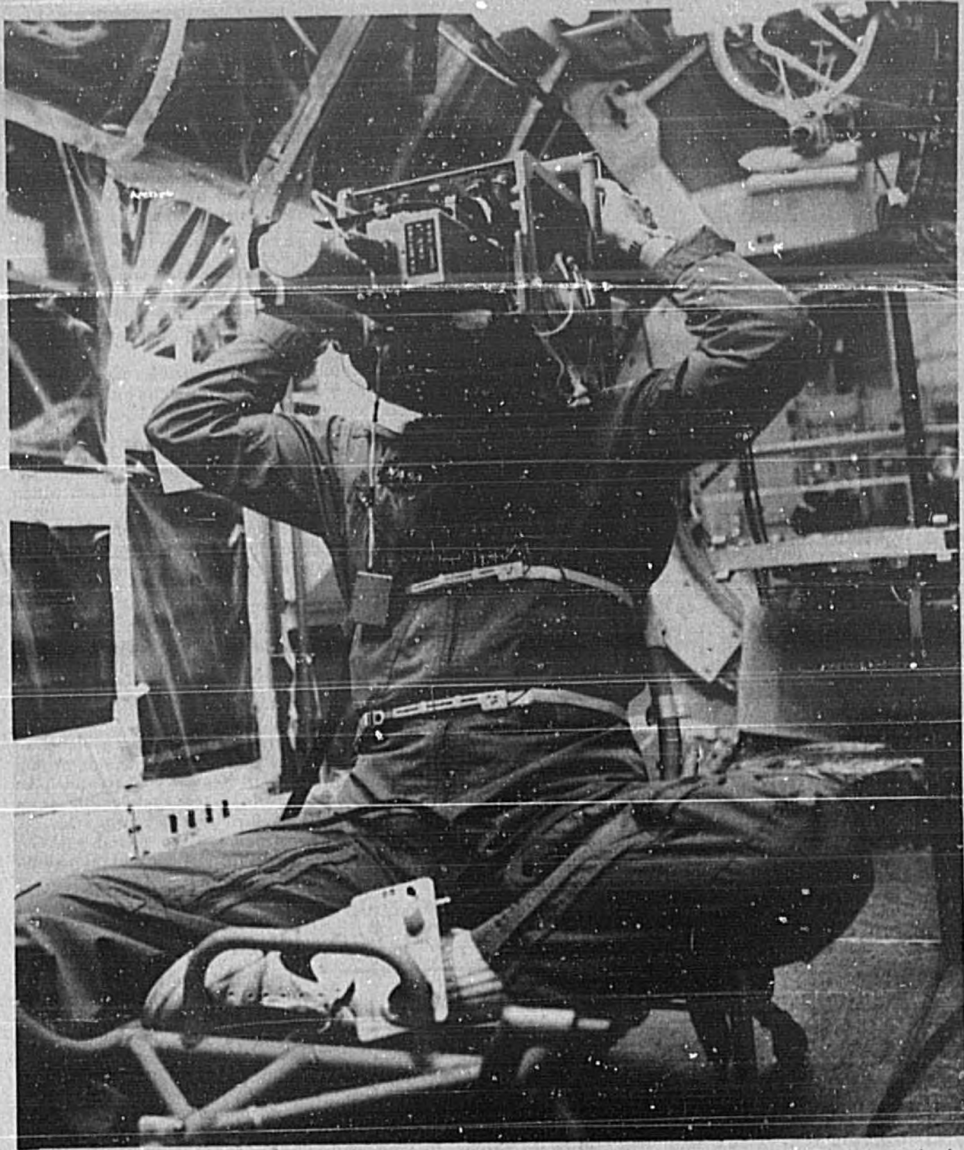
Spacelab mission specialist Robert Parker wears a device that measures eye movements during investigations to determine how the human body reacts to space. The chair and sensor package is subtle body motions under weightlessness. The experiment will be part of spacelab's series of habitable module.
