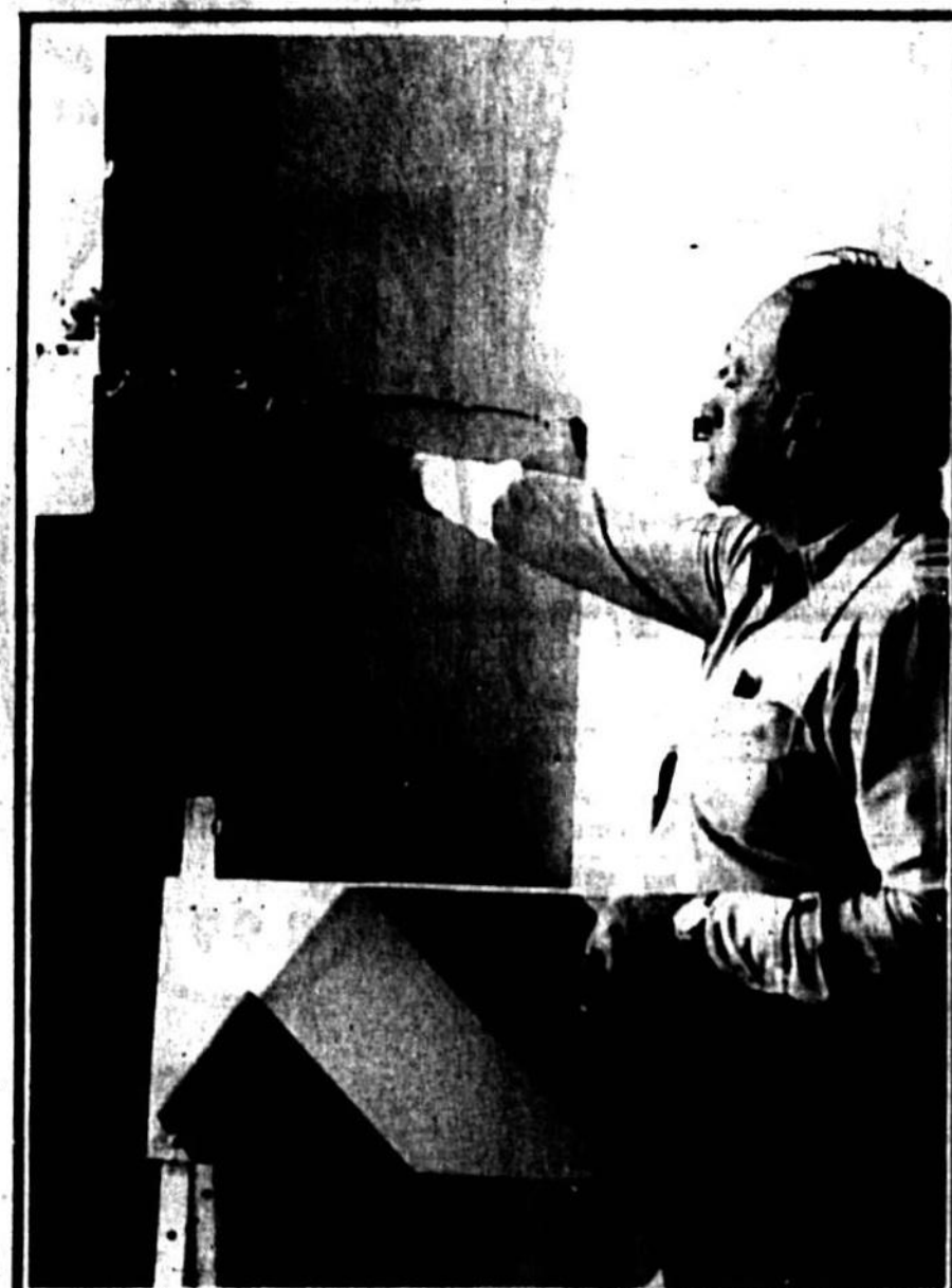
A CRACK OFF THE OLD BLOCK City Building Official Frank Boyles points to crack in column in front of Casselberry City Hall damaged by windstorm Sunday afternoon. The city's insurance company is still getting estimates from contractors for removing and replacing the damaged column, City Clerk Mary Hawthorne said today.
