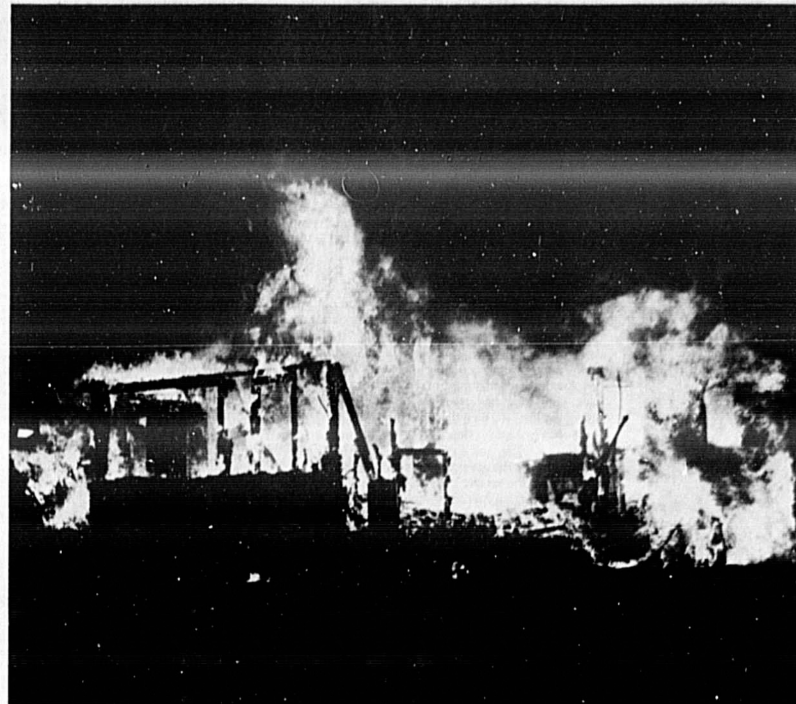
HEATER FIRE DESTROYS HOUSE An oil heater exploded and flames destroyed a five room frame house in the 2200 block of Alexander Avenue, Sanford, Saturday night. Lawrence Williams told authorities he, his wife, Frances Hall and the home owner, Ella Mae Hall barely escaped, as flames raced through the house after the explosion. The house was destroyed before Lake Mary Volunteer Firemen could respond to the densely populated area east of Airport Boulevard and north of Country Club Road, but firemen wet down surrounding structures and kept the fire from spreading. (Bill Vincent Photo)
