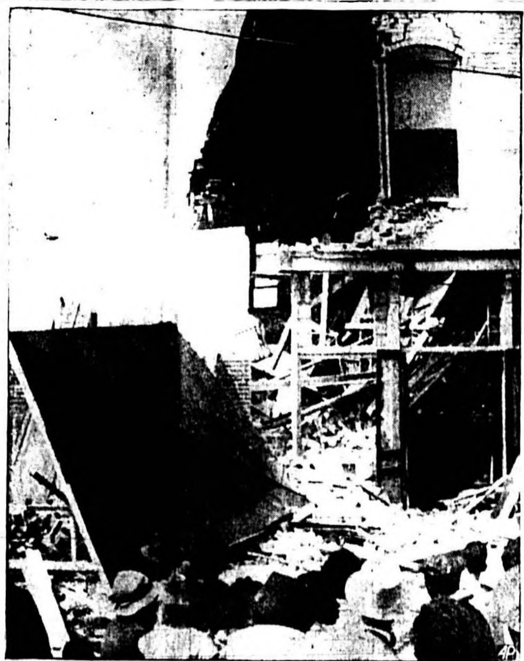
In this shambles, all that remains of a building that collapsed in the business section of the City, Ala. 11 men died and 26 others were injured, enough to require hospital treatment.
