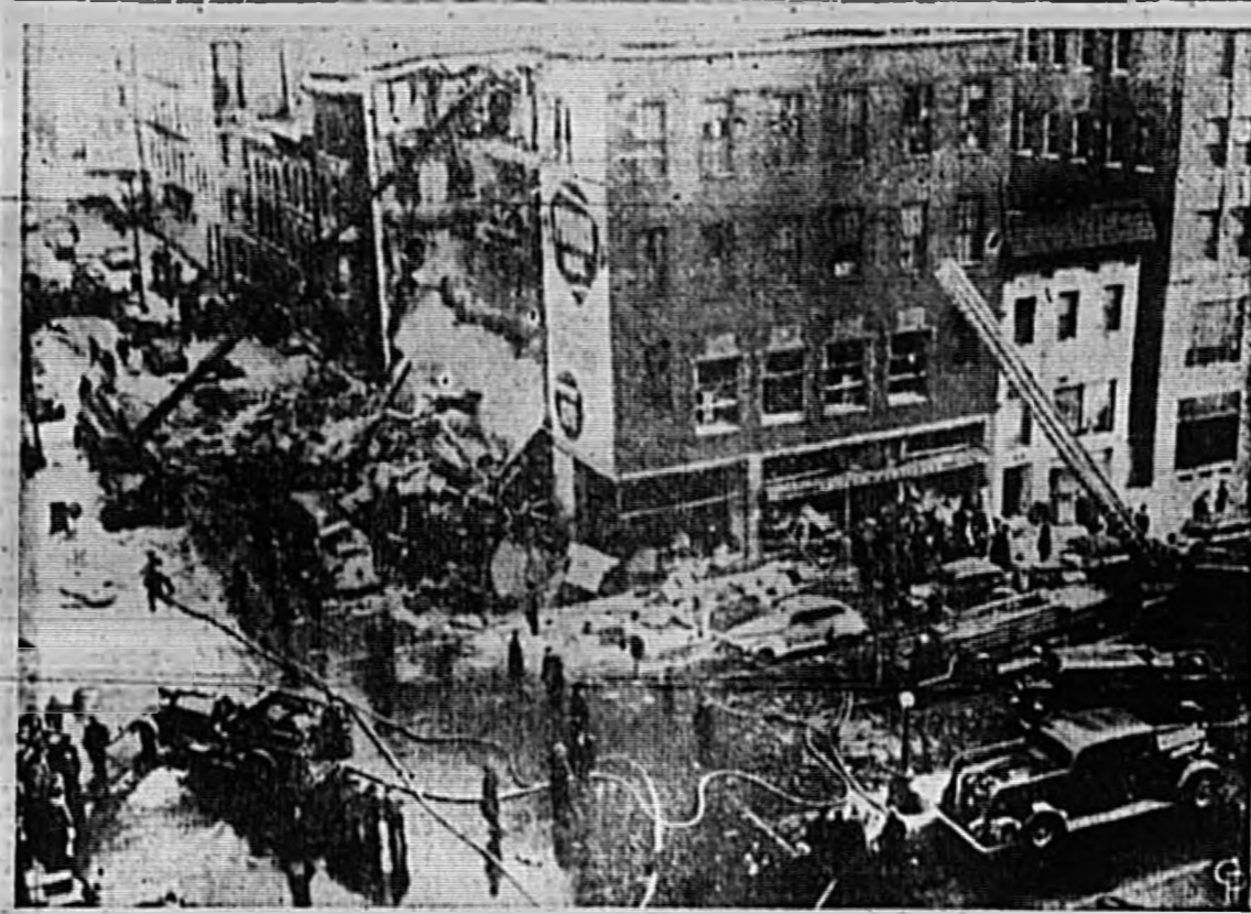
FIVE PERSONS WERE KILLED and six injured when an explosion blew out a complete wall of this four-story furniture building in Chicago. The blast occurred shortly after a company employee reported a gas leak. Cars parked near the wrecked structure were shattered by pieces of household articles. (International)
