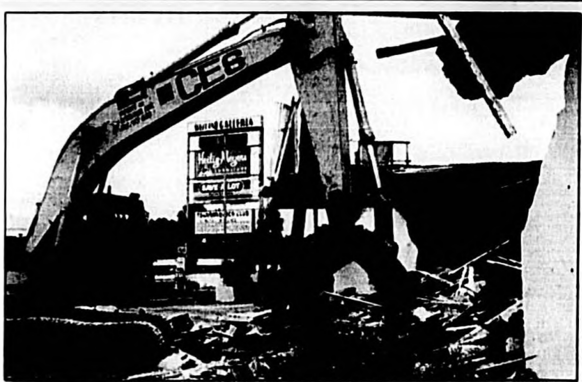
Demolition crews demolished a building at the West End Galleria in Sanford to make way for the upcoming GreeneWay expansion that will connect the northeast portion of Seminole County to Interstate 4.
